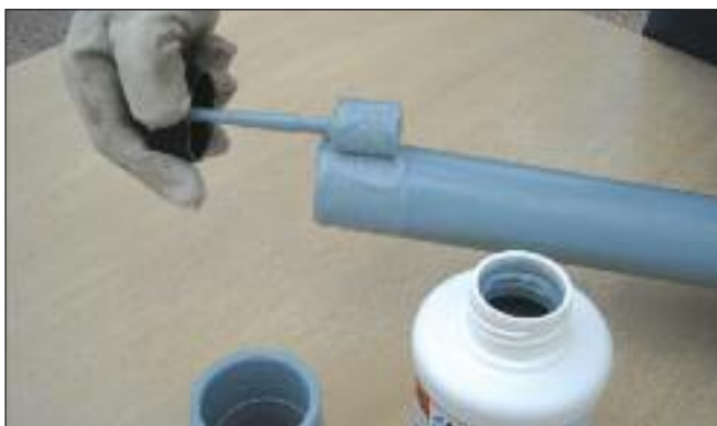
9. Apply cement to pipe and fitting.
